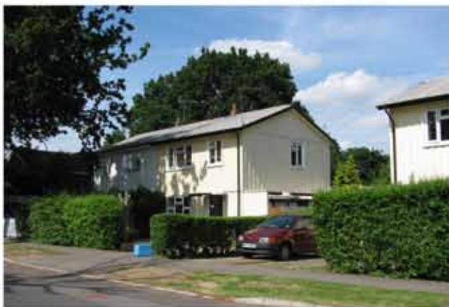
Airey Homes on Mayfield Road – prefabricated construction in the post-war period
