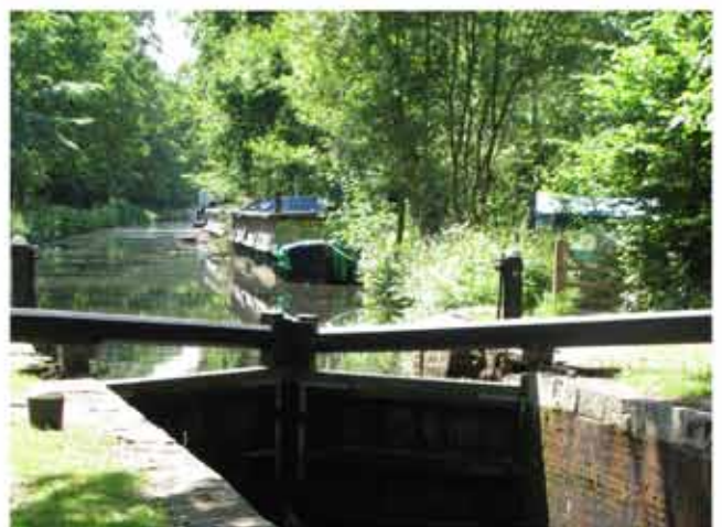
The Basingstoke Canal at Scotland Bridge – a visually and physically important element of the local character
