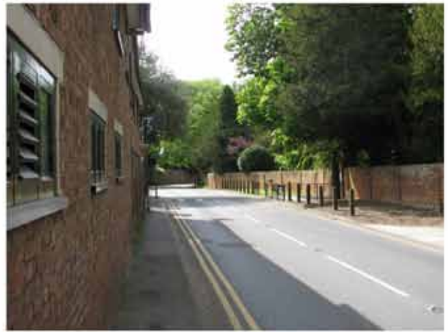
High brick boundary walls adjoining the roads add to local distinctiveness and character in the Thorpe Village Conservation Area
