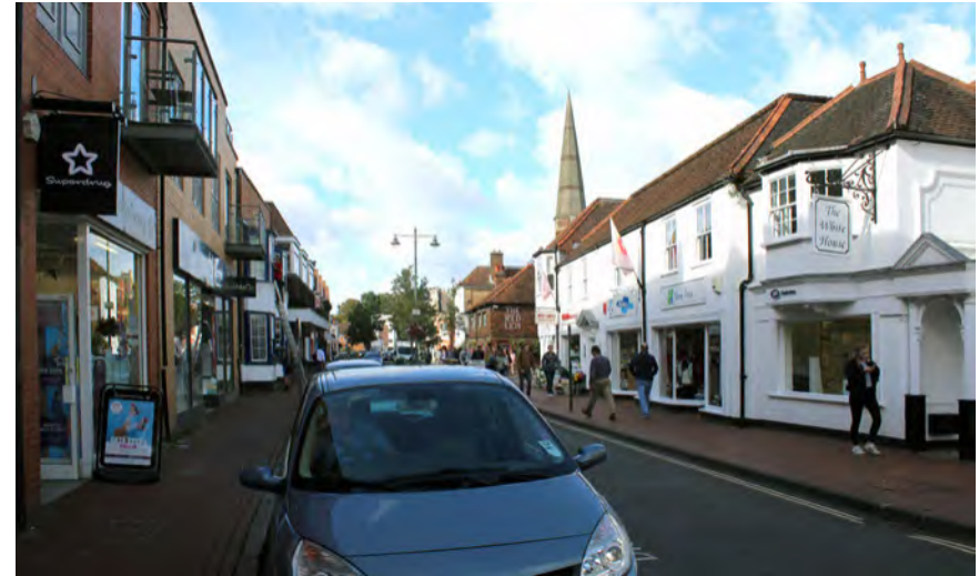
View along the High Street showing the buildings hard against the pavement edge
