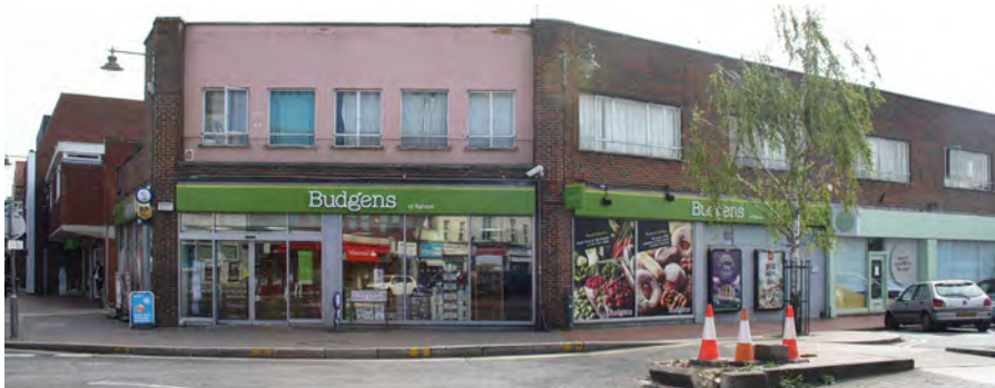
Nos. 1-11 Station Road North, detracting building
