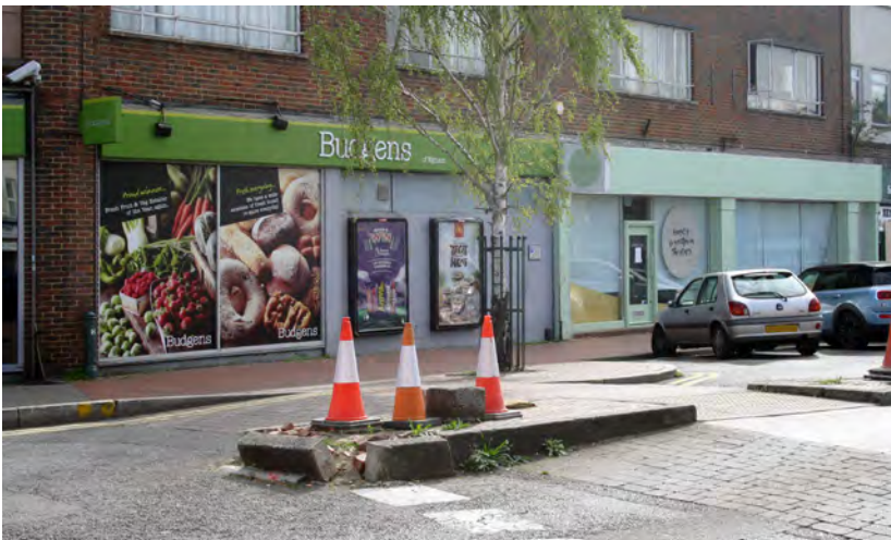
Damage to surface treatments at junction of High Street and Station Road North
