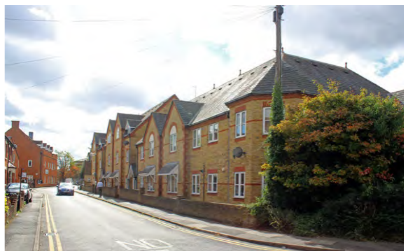
Hummer Road looking south-west
