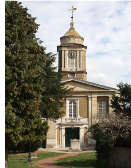
St John the Baptist's Church, Grade II* listed
