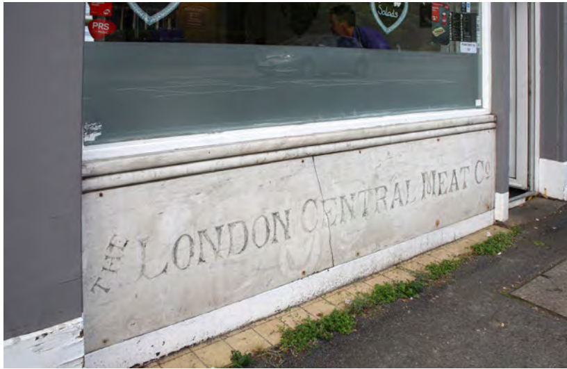
Shopfront and marble signage of No. 176 High Street
