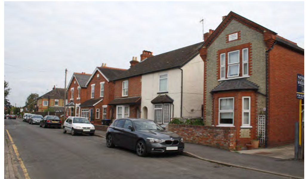
Residential houses in Crown Road in which the windows have been converted to uPVC
