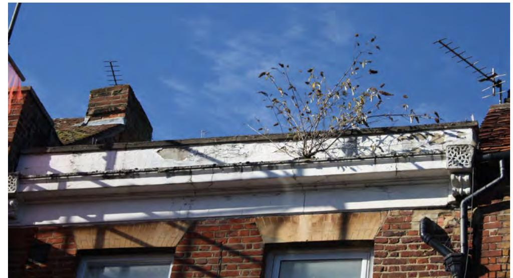
*Examples of peeling paintwork, foliage growth and rotting timber, all of which are preventable through routine maintenance*
