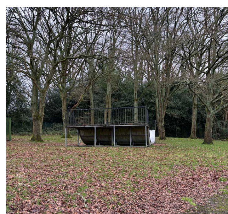
View of the existing skate ramp
