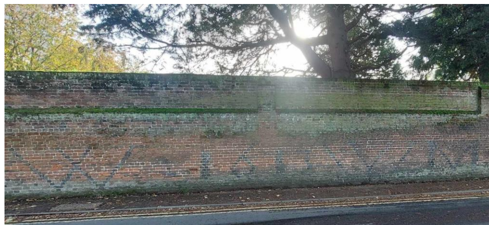
Figure 7: Diaper brickwork in the boundary wall on the south of Coldharbour Lane, spelling W 1613 W M.
