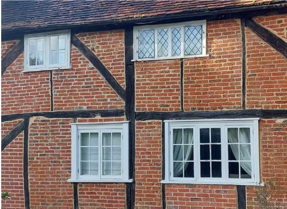
Figure 29: Timber-framed casement windows.
