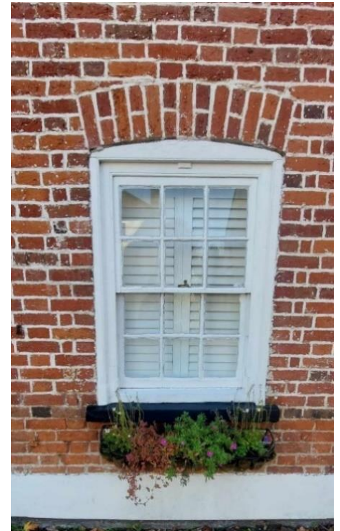
Figure 28: A square headed, timber-framed sash window with brick detailing above.
