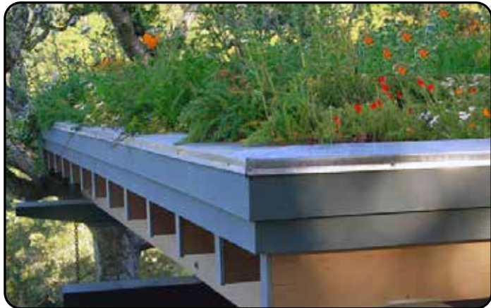
Favour ease of maintenance and accessibility to the green roof
