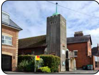
2. Methodist church, Listed Grade II
