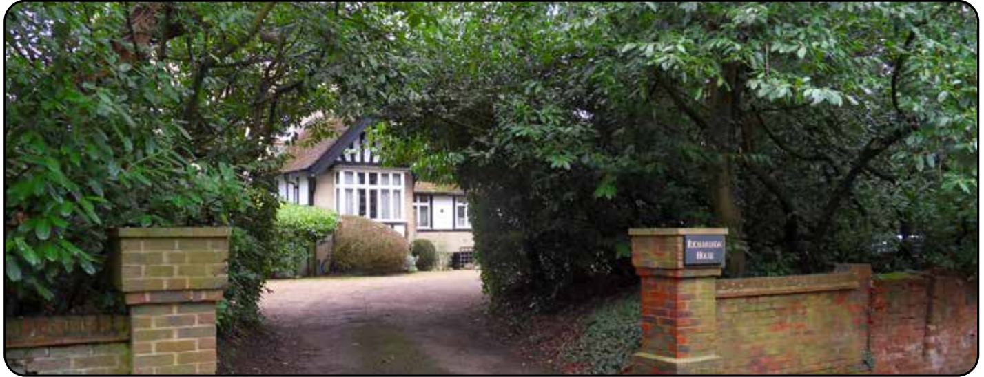
Cooper's Hill Lane. View of Richardson House, exemplary of the type of bigger properties in the open land
