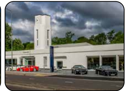
15. Tower Garage, Listed Grade II
