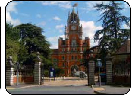
5. Royal Holloway Entrance Gates, Listed Grade II
