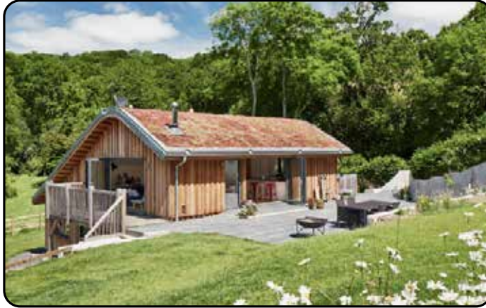
Protect green roofs and walls from excessive wind levels, in this case the sloping site assists in the protection of the roof
