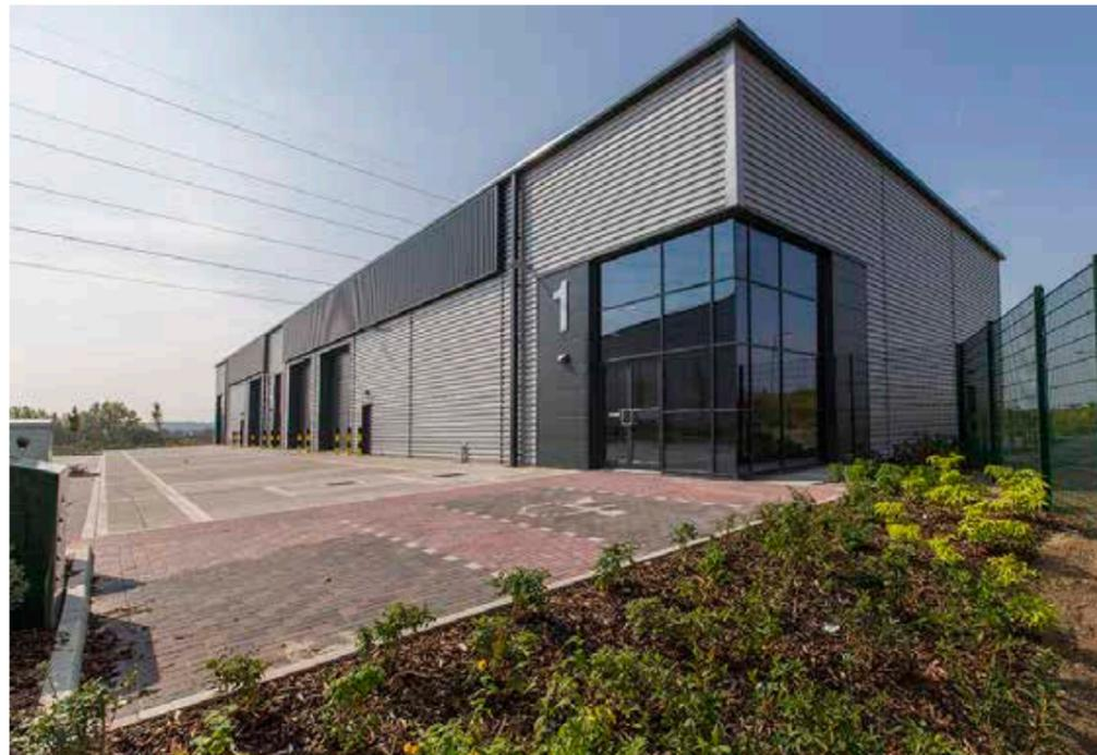
Photograph of the industrial unit illustrates the type of metal cladding combinations that are available
