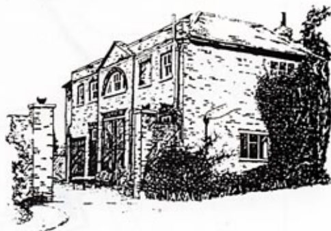
The 'thermal' windows (derived from classical Roman architecture) are a particularly nice feature of this 18th century building. It was originally the stable block to Englefield Green House, and was later converted to a coach house (as shown here). The coach house doors have now been replaced with windows.
