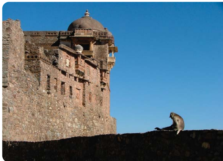
Jaisalmer Fort, Rajasthan
